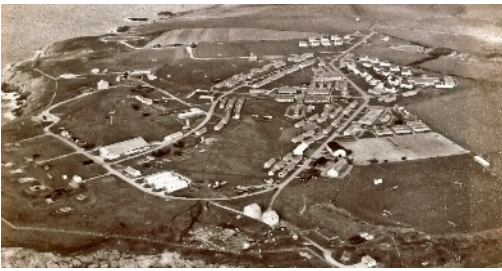
Aerial picture of the MOD camp
